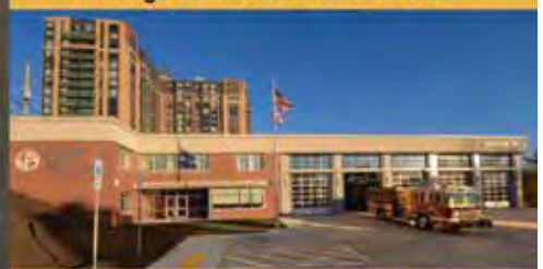
Towson Fire Station No. 1
